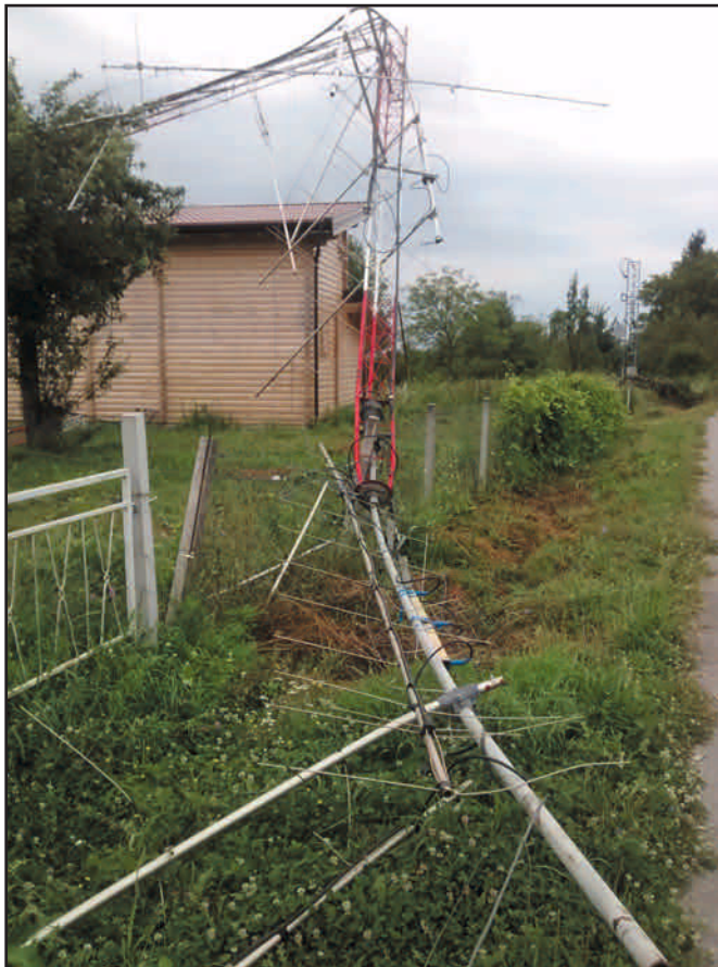
The 100-foot tower of 9A9R, the top band score from Europe, was destroyed by a tornado shortly after the contest.
